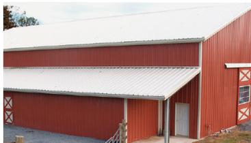
AZ 55 Galvalume is used for Ironbuilt's roof coating. It is composed of a 55% aluminum, 43% zinc, and 2% silicon. The aluminum and silicon combine to produce a barrier to corrosion. Galvalume is maintenance free, requires no painting and keeps its original sheen.
