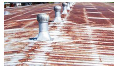
Most companies use AZ 50 Galvalume coating on their roof panels which has a thinner coating than Ironbuilt's roof. Since it is not as effective as Ironbuilt's coating, only a 20 year warranty is offered. Other companies use only a regular galvanized coating which is prone to rusting and perforations that cause leaks.
